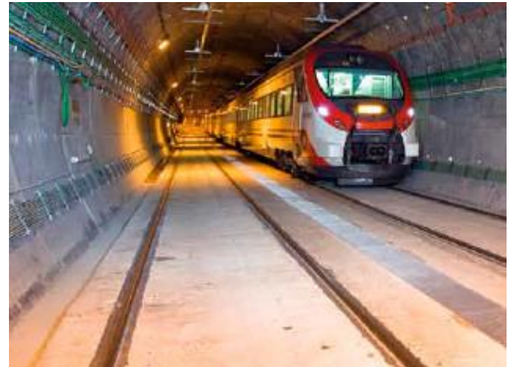
Embedded Rail System (ERS – Edilon)(Sedra )
